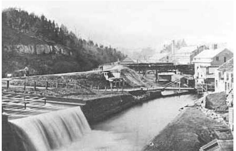
Upper Raceway with spillway into Middle Raceway in the 1800's
